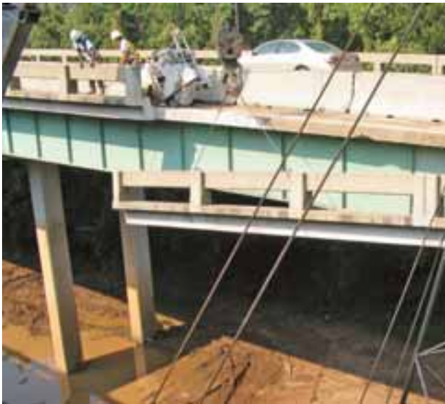
Dawson Bridge rail removal in Montgomery
